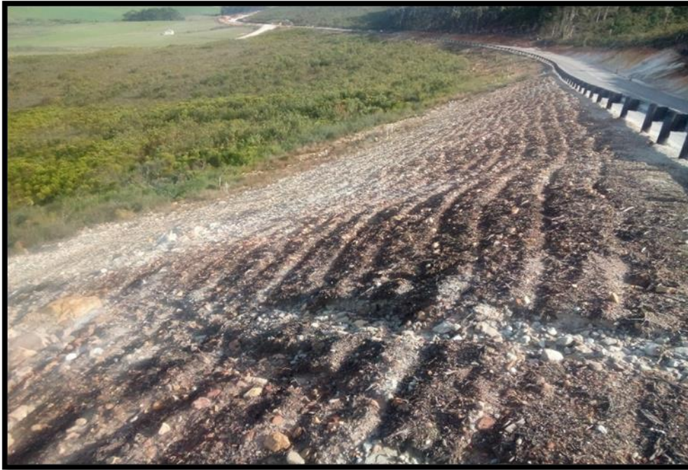
Figure 9: Example of horizontal terracing to reduce down slope erosion.
