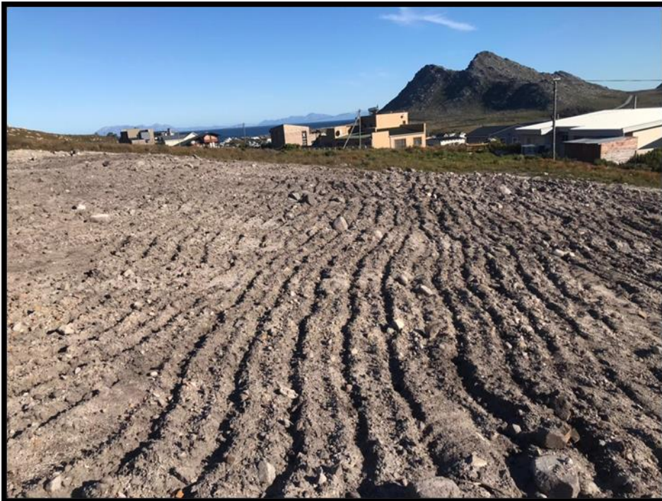
Figure 8: Example of a previously compacted area that has been ripped, shaped and topsoil spread over the affected area prior to rehabilitation.
