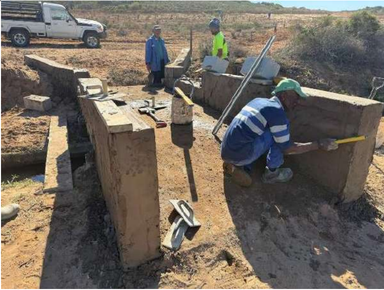
Photo 4: Stormwater overpasses are being constructed over the irrigation canal as per the instructions in the Stormwater Management Plan, to prevent damage to the canal during times of heavy rains.
