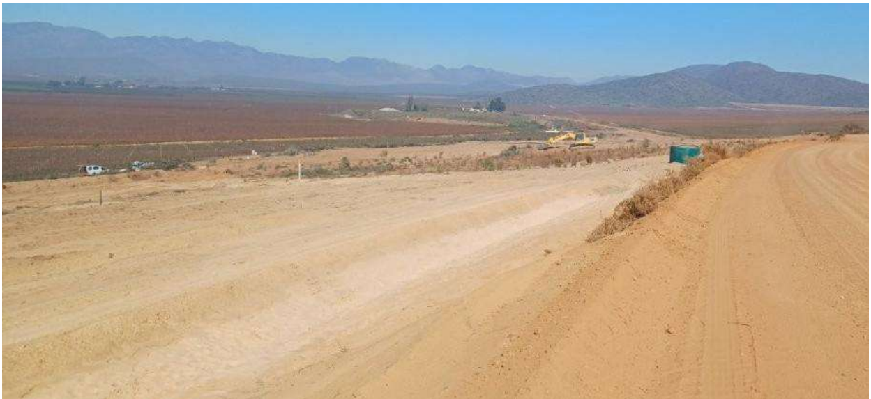
Photo 1: The area that was wrongfully cleared within Cultivation Area 2 can be observed in the foreground, left of the road.
