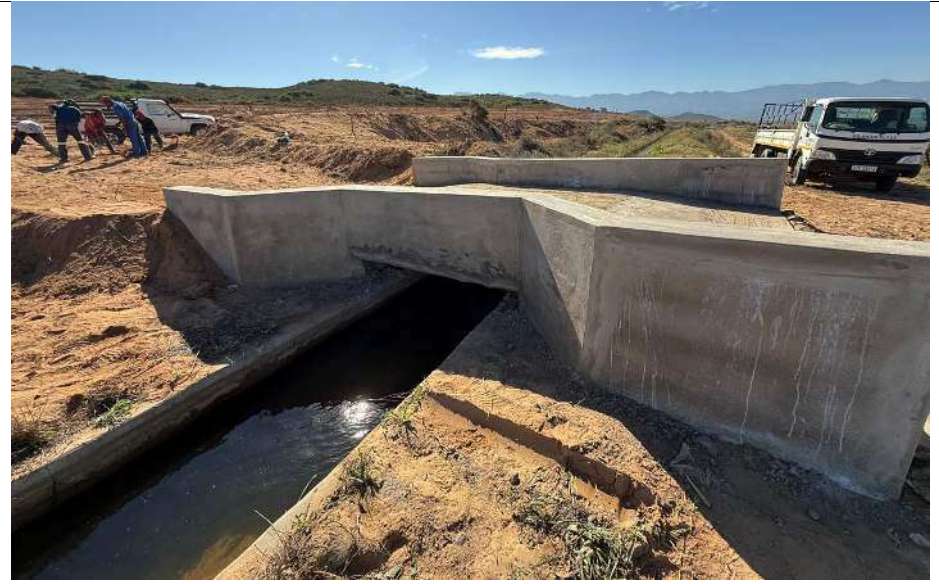
Photo 5: A completed stormwater overpass, constructed according to the directions of the Stormwater Management Plan.
