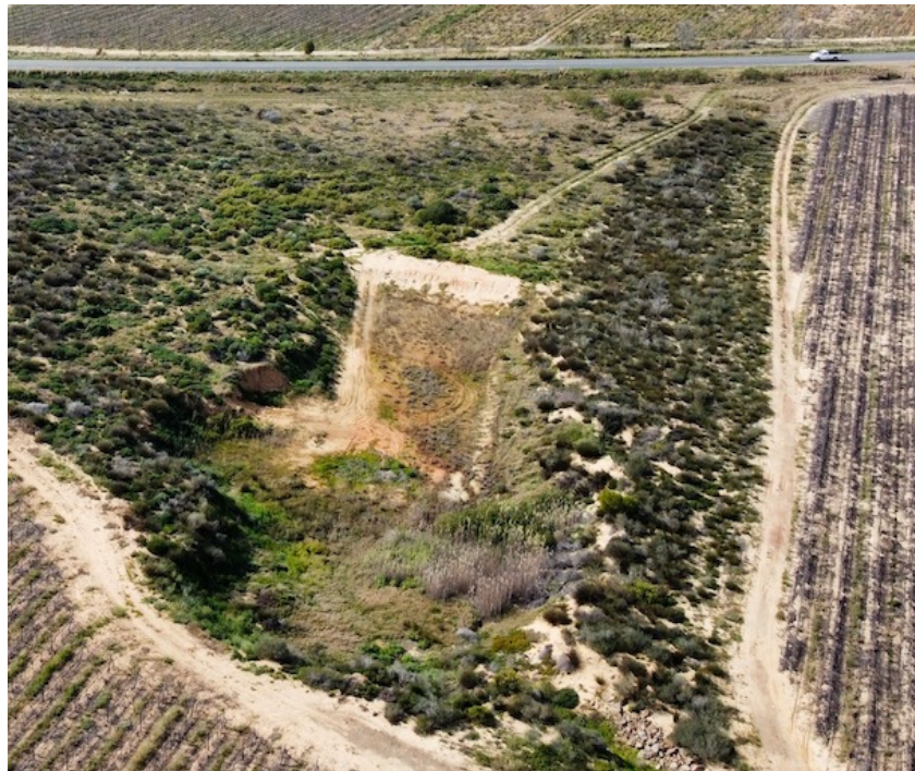
FIGURE 3: ATTENUATION DAM WHICH RECEIVES RUNOFF FROM AREAS C6 AND C7
