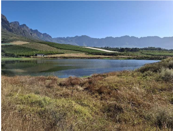
Figure 8: Looking east across the dam.
