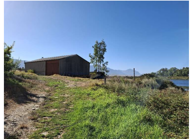
Figure 18: This shed may be affected by the new enlarged dam basin.
