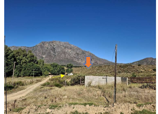
Figure 3: Looking west towards the pumpstation and southern section of the dam wall. Pump station marked by yellow arrow.
