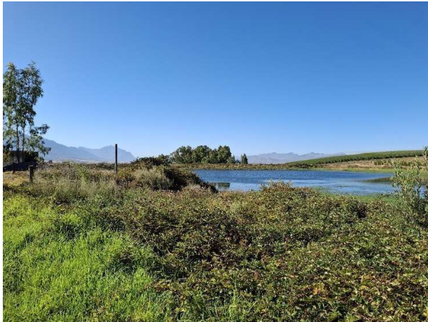
Figure 17: Looking south across the eastern portion of the dam.
