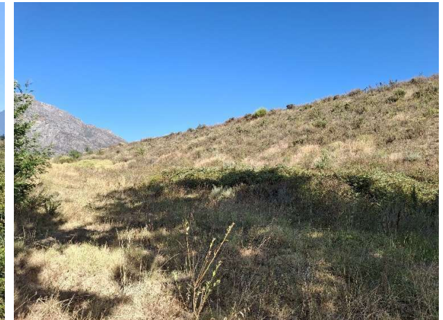
Figure 6: The dam embankment which will be increased to accommodate the expansion.
