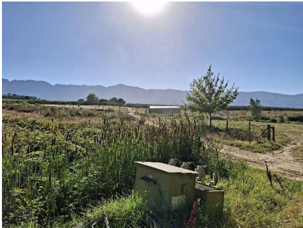
Figure 4: Downstream of the dam wall.
