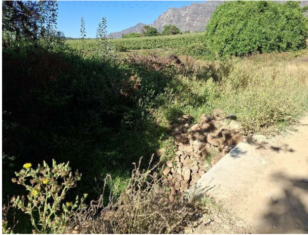
Figure 20: The piped section of the watercourse entering the dam.
