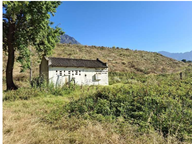
Figure 5: The pumpstation below the dam wall.
