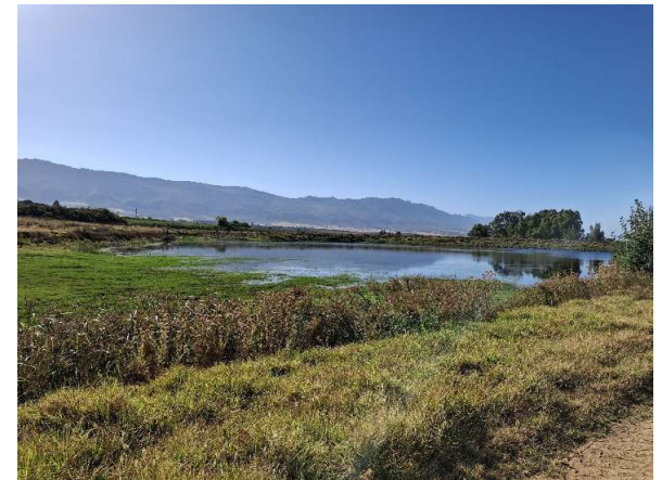
Figure 12: Looking south across the dam.
