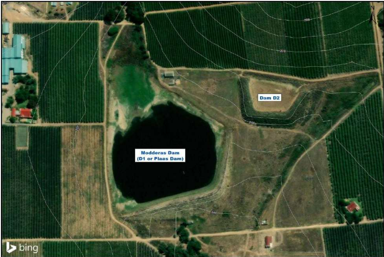
Figure 2-1: Existing dams on Farm 1/66
