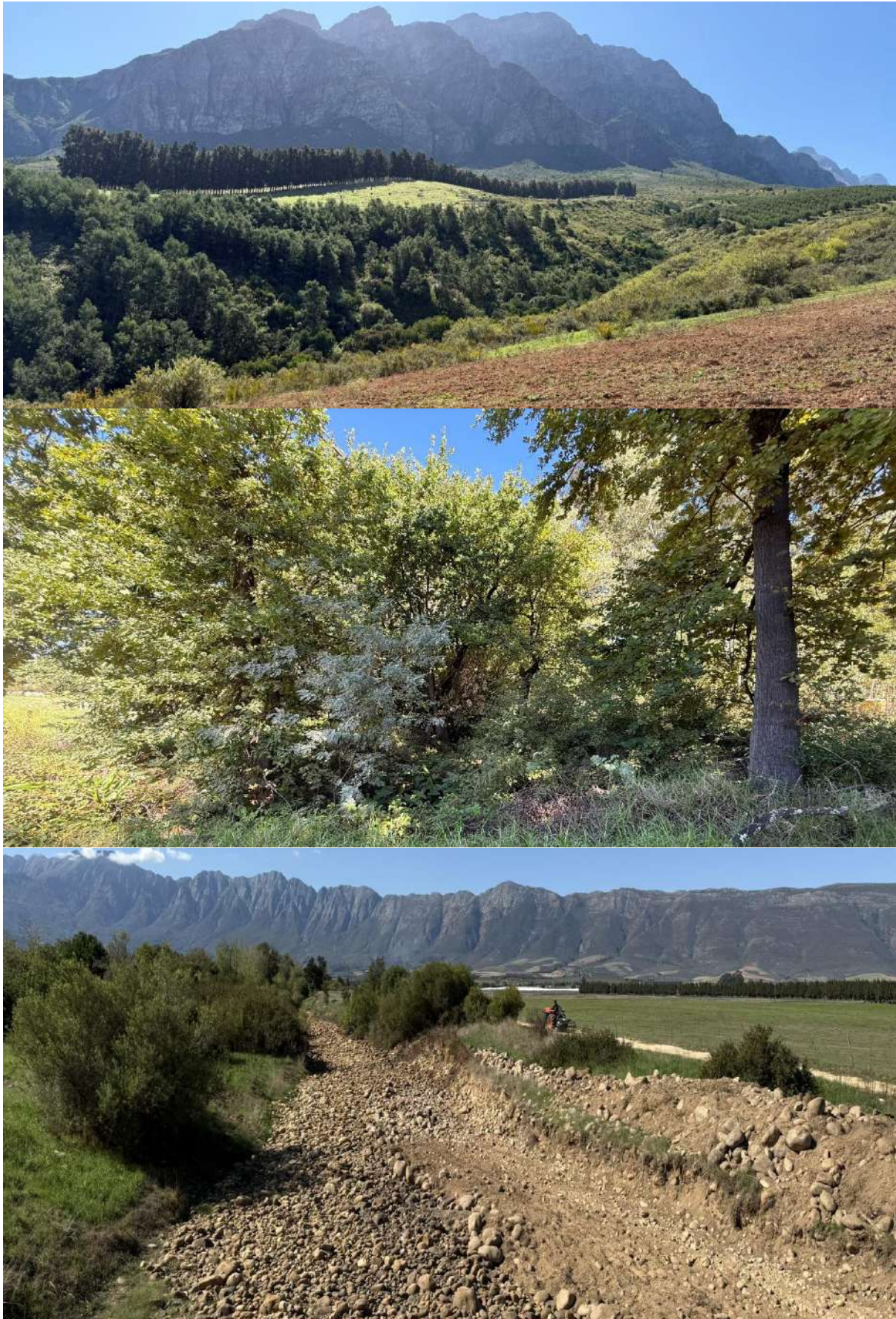
Figure 10. Views of the Modderas Stream upstream (top and centre) and downstream (bottom) of the dam
