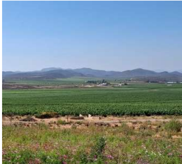
Stormwater Management – Stormwater overpasses have been constructed to protect the irrigation canal.
