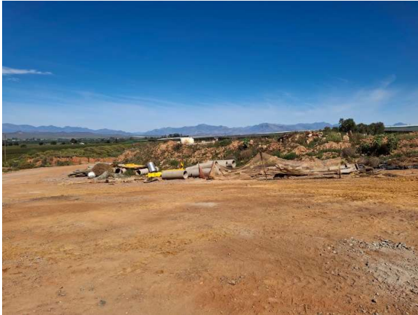
Excess materials should be stored in a demarcated waste area.
