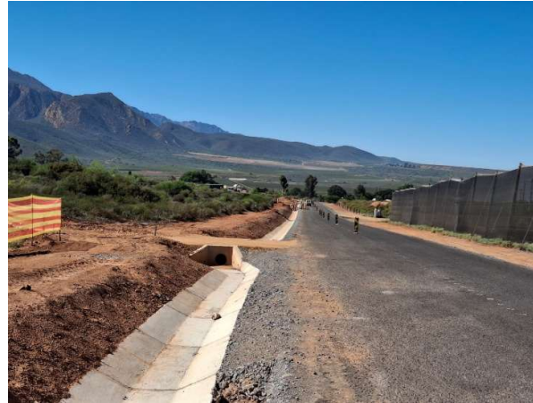
Access points provided to neighbouring farms with stormwater control in place.
