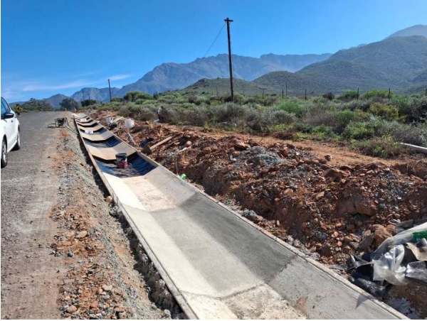
Activities underway along this section of the stormwater channels.
