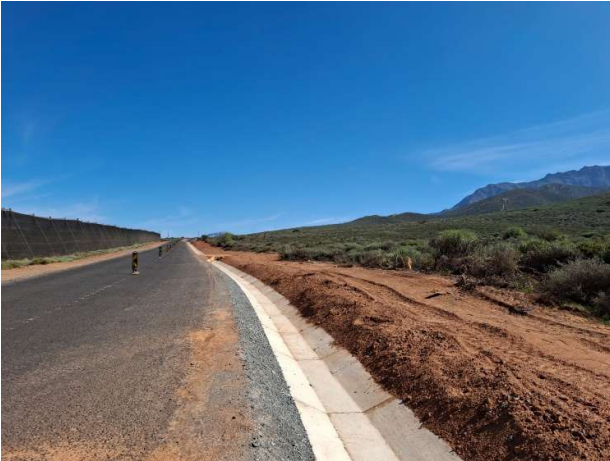
Stormwater drains/channels complete towards the mind section of the road.
