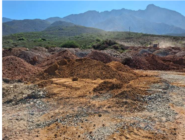
Stockpiles within the laydown area.
